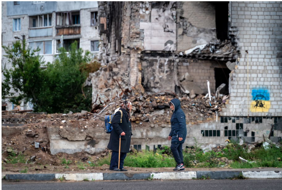
Two residents of Borodianka, Kyiv region, next to a damaged building. Photo: OCHA/Matteo Minasi
